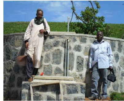
Edwin Visi, our consultant engineer and a villager near a finished storage tank.
